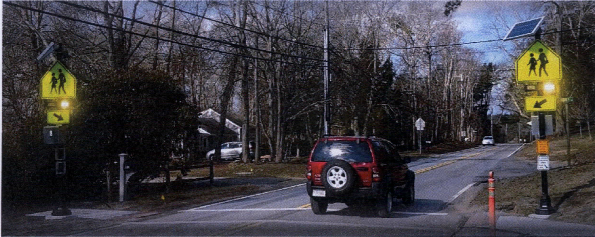
Figure 1 - Gate-posted RRFB installation at a school crosswalk
